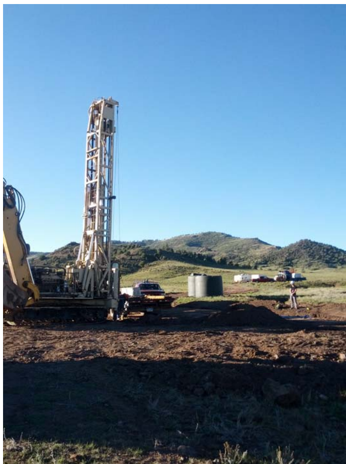
Figure 3 – Drilling water monitoring wells at the Hansen Deposit, November 2013.
